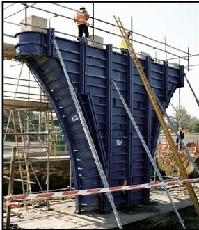
These moulds can be long and difficult to set up and take a long time to demould, but will generally last the test of time due to their extremely good durability.
